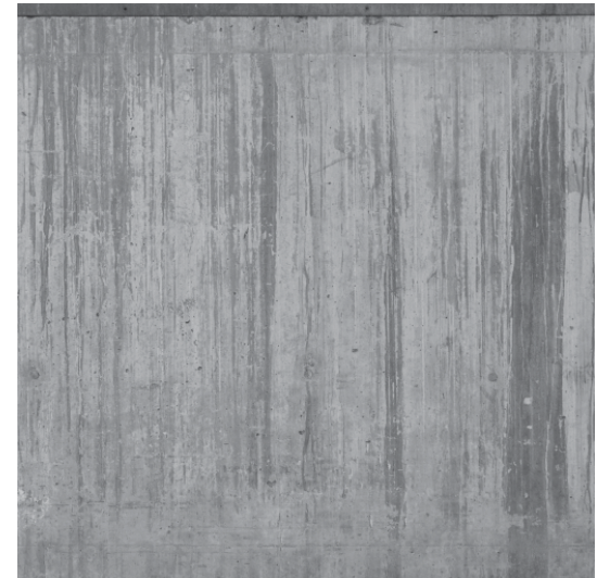
Concrete wall photograph
